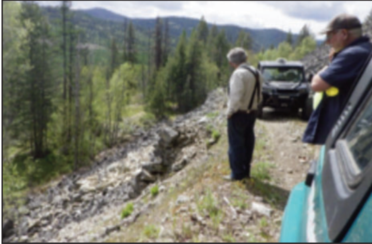
Bob and Dave checking out the hand stacked rocks supporting the Franklin Heritage Trail. There is over 600 feet of stacked rocks, most vertical. How— who did it?
